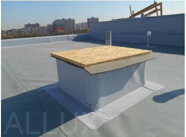
Before the actual installation of the roof part of the ALLUX light tunnel, cover the base to protect it from rain so that the mineral wool inside the base does not get wet.
