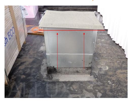
Pull the steamproof film on the external side of the base as high as possible to the top edge of the base.
