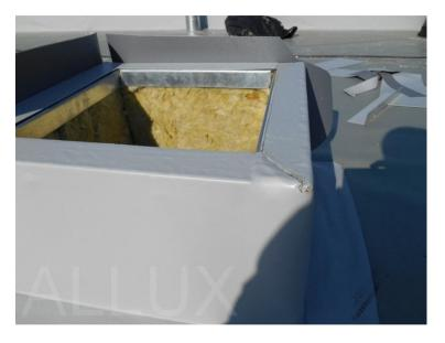
Check that the waterproofing is properly melted to the upper edge of the base and there are not air gaps anywhere.
